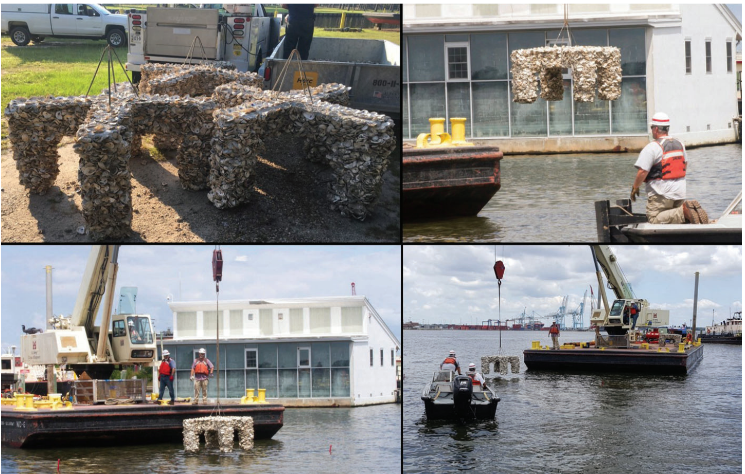
3 ft tall X-Reefs being deployed in Fort Norfolk. Photo courtesy of Russell Burke.
